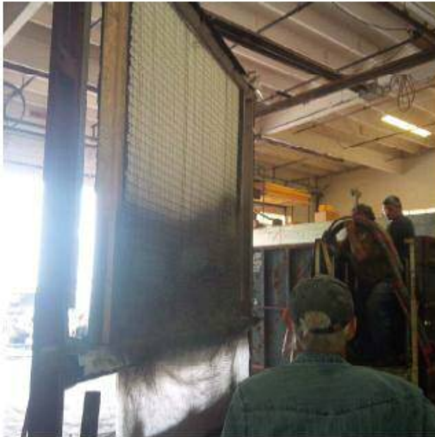
Photo 7. Schnell Wire Systems s.r.l. Test Wall Sample Concrete Application
