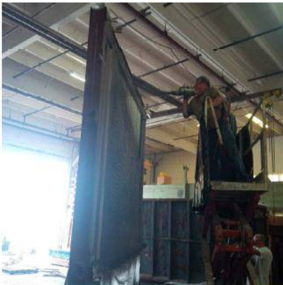
Photo 8. Schnell Wire Systems s.r.l. Test Wall Sample Concrete Application
