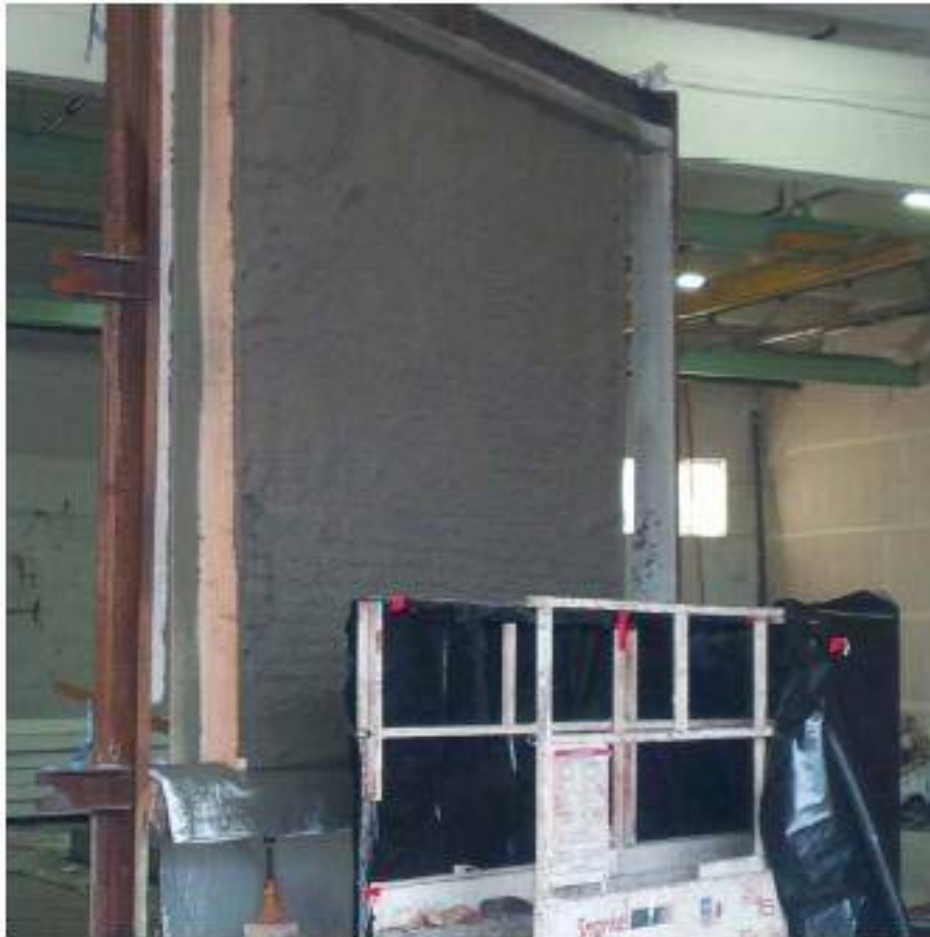
Photo 10. Schnell Wire Systems s.r.l. Finished Test Wall
