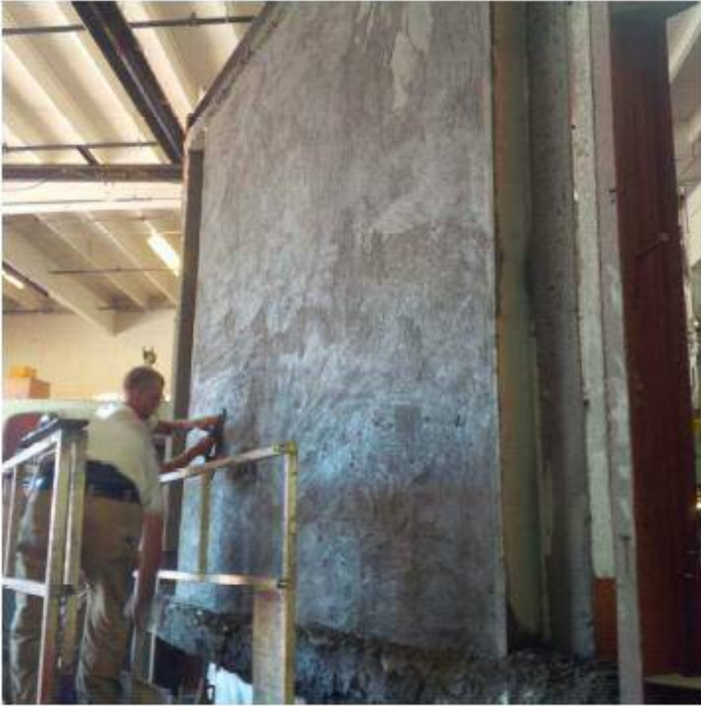
Photo 9. Schnell Wire Systems s.r.l. Test Wall Sample Finishing
